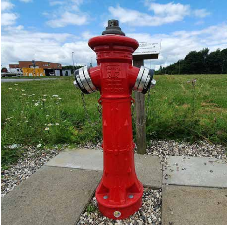
Hydrant with VIDI Caps installed. The use of a hydrant affects the pressure in an area. Therefore, it is important for the utility to know when the hydrant is being used in order to distinguish between a pressure drop coming from regular use or from a pipe burst.
